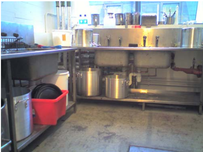
The Dye lab is used for mixing, heating and disposing dyes. It has burners to heat the dyes, along with sinks to wash off dyes. The dye lab does not have dedicated heating systems, but does have hot water delivery pipes for the underfloor heating system in the print room running under the sink on two adjacent walls.
